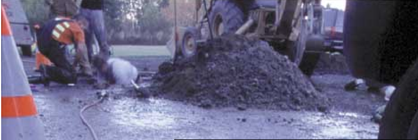
(Left) Water Main Repair - Gig Harbor, WA
